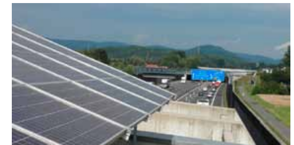
solartunnel Hosbach, Frankfurt
